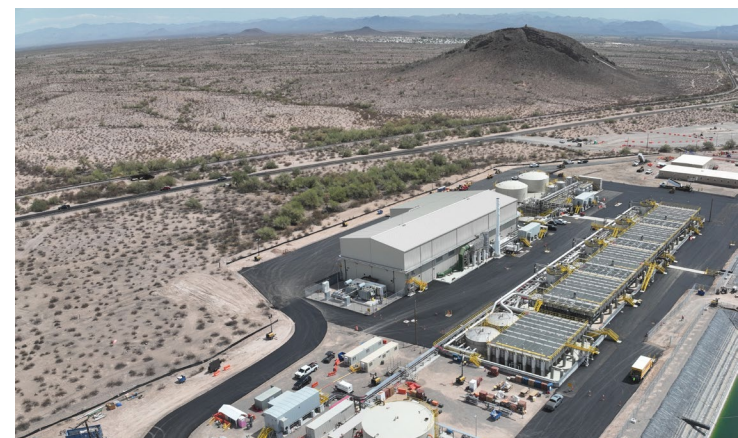
▲ Construction of Florence Copper facility
